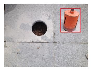
.... often making it easier to lift the slab/s ..... if no access to core drill a neatly cut corner section is an alternative option - using an angle grinder
