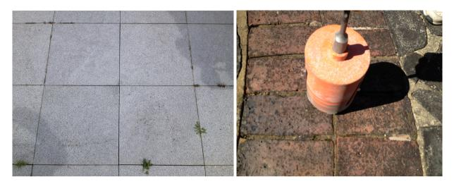
2 Core drill the slab at required position
