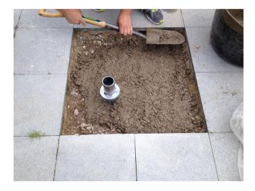
7 Ensure that socket is absolutely vertical with spirit level ... and that the point where the two widest diameter plates join is level with the FINISHED surface
